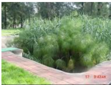
Fig. 7a. UNAM Coyoacán Vivarium subsuperficial horizontal flow artificial wetland (23)
