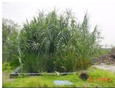
Fig. 7b. UNAM Cultural Zone subsuperficial descending vertical flow artificial wetland (23)
